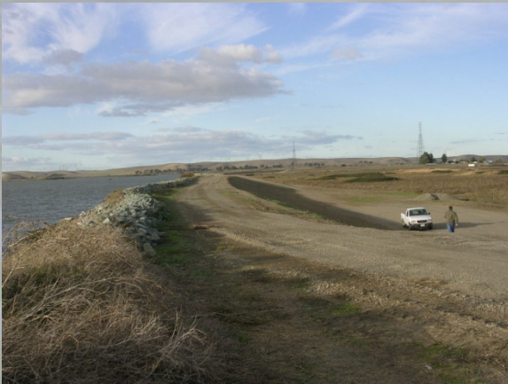
Conditions of Mayberry Slough Levee prior to construction
