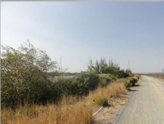
Mayberry Slough Levee in 2012, after construction and AB 360 inspection
