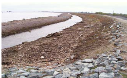
Setback Levee on Twitchell prior to vegetation growth
