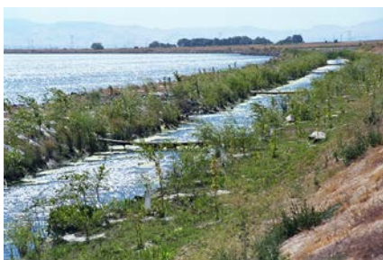
Plant growth is evident one year after the setback construction
