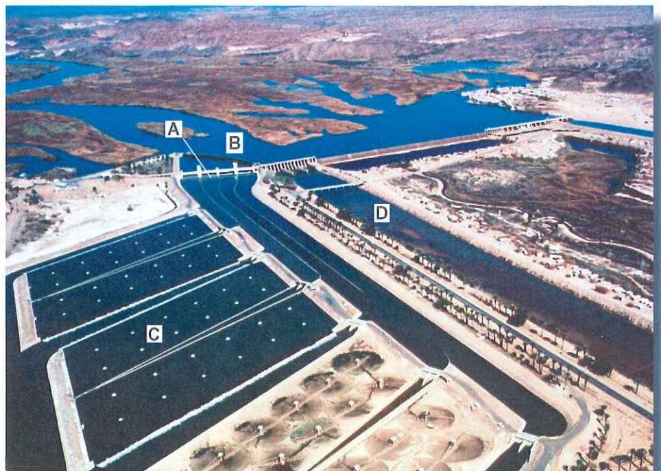
This Bureau photo shows: (A) Imperial Dam; (B) trashracks; (C) the three desilting basins; and (D) the California Sluiceway.
