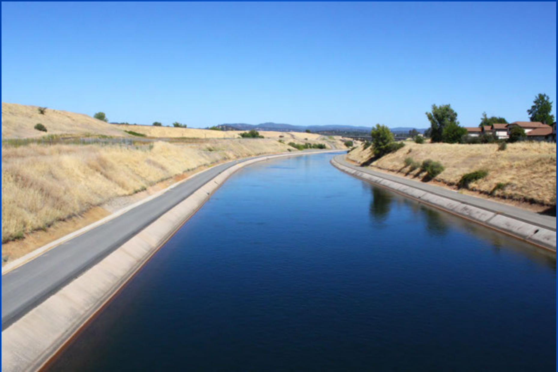
The Thermalito Power Canal delivers the diverted water to the Thermalito Forebay.
