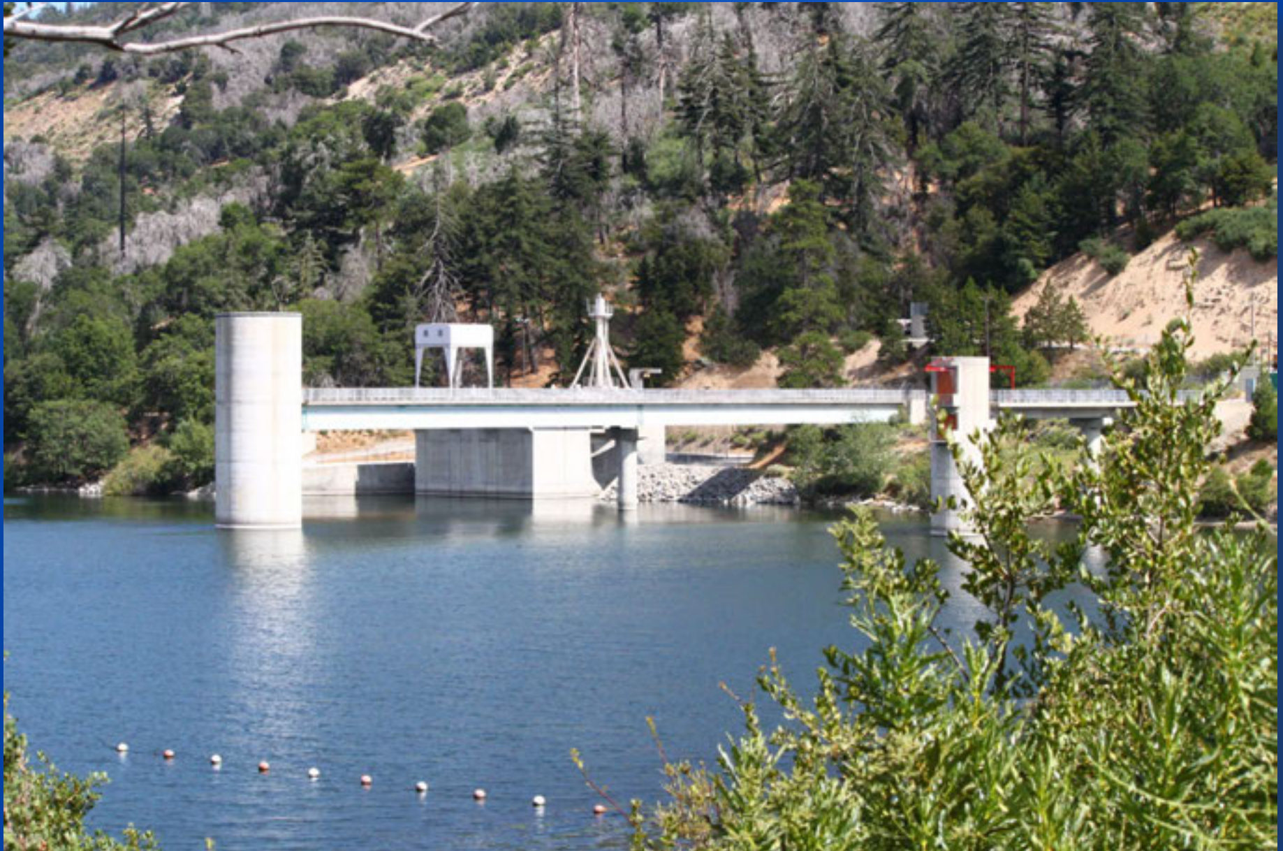
The water leaves Silverwood Lake and enters the four-mile long San Bernardino Tunnel.
