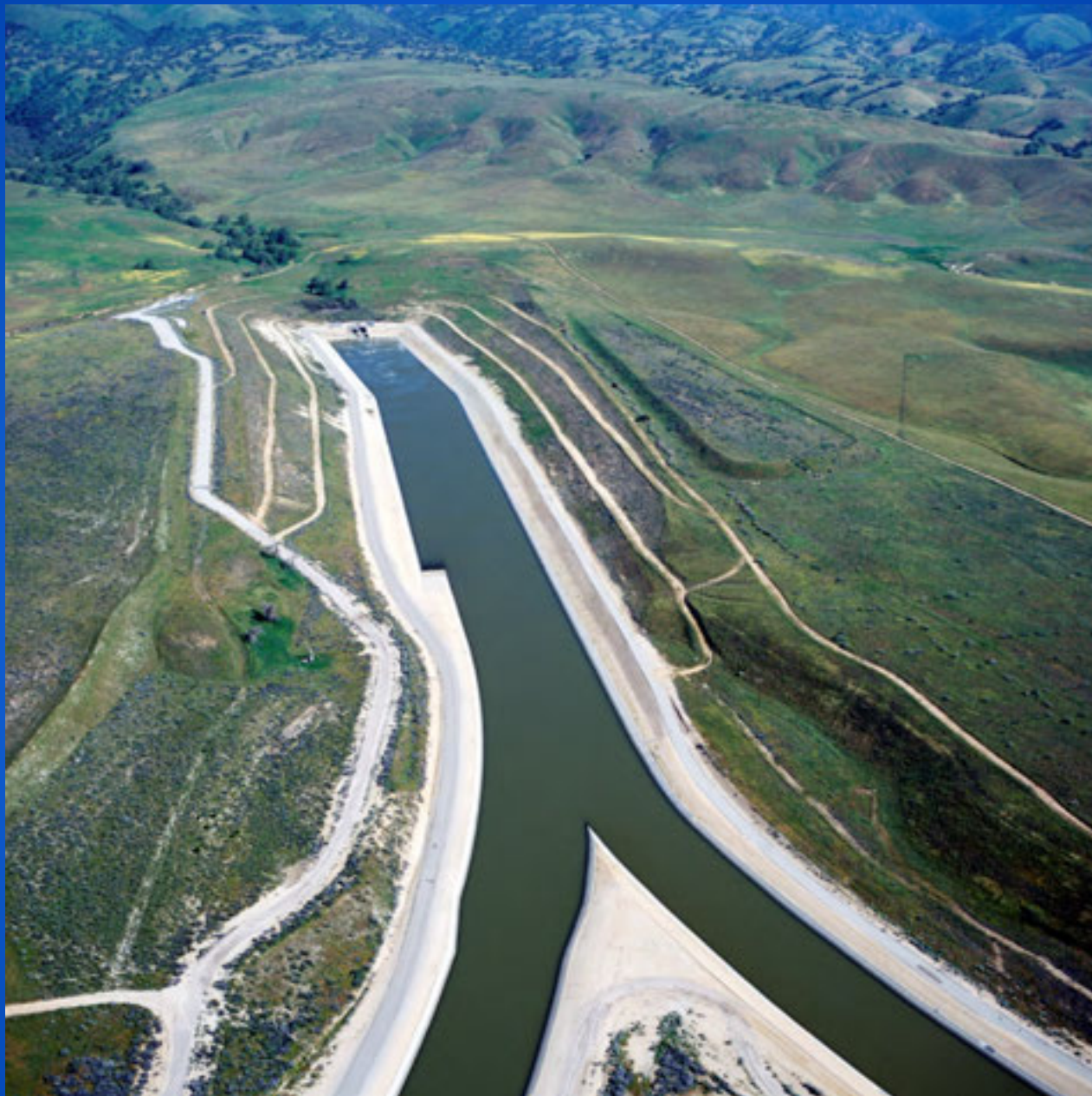
Once the water reaches the top of the Tehachapi Mountains, the aqueduct splits into the East Branch and the West Branch.
